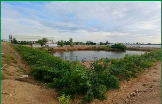
Rainwater harvesting ponds: ~ 61,000 KL
