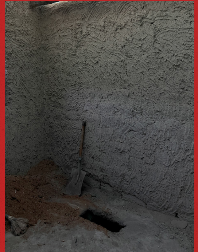
Dry compost toilet in Chilling.
