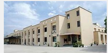
Eicher Engineering Component – Dewas
